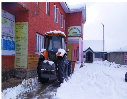
Photo 3: Restoration of Road linkages of Health Services facilities has to be the Priority
