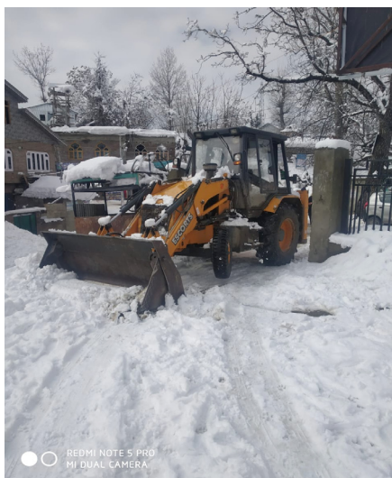
Photo 9: MED men and machinery busy in Snow clearance in Srinagar
