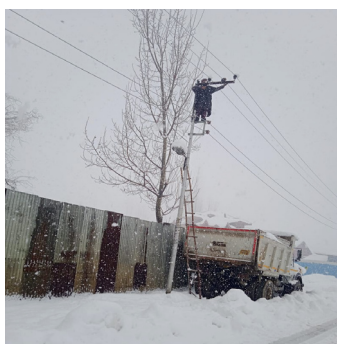
Photo 5: Restoration of Power Supply
