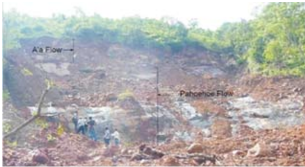
Figure 12: Basaltic rock exposed in 4 th Zone bottomed
