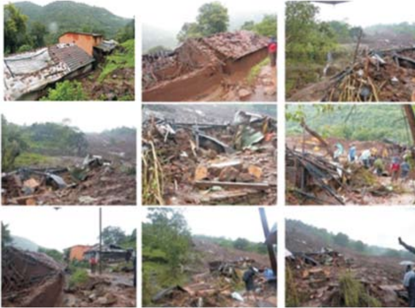
Figure 24: Complete Damage to houses due to movement of debris material
