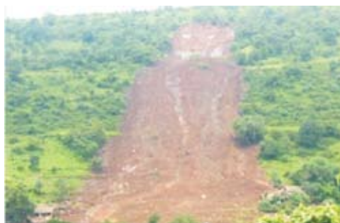
Figure 13: Gullies within the slided zone
