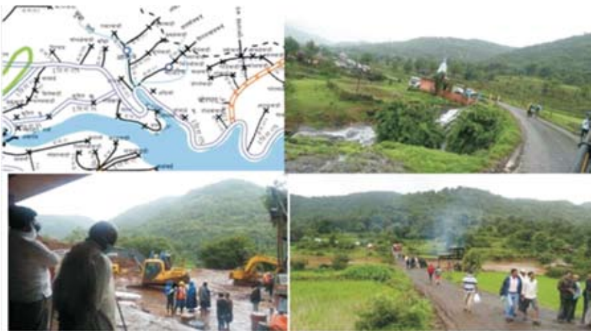
Figure 22: Road constructed under the various schemes at Malin village
