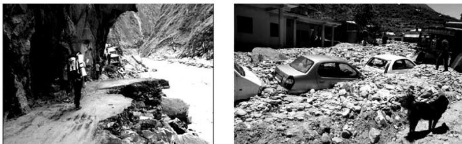
Fig. 4 View of road disruption in June, 2013 due to bank erosion in the proximity of Tawaghat, Pithoragarh (left) and debris slide in Dharali, Uttarkashi (right)
