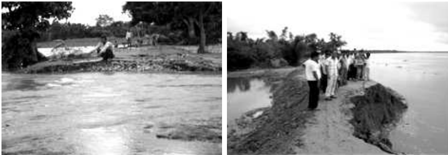
Fig 5: Breach and river erosion on the bank of river Bharamputra (Source: DM Office, Barpeta)
