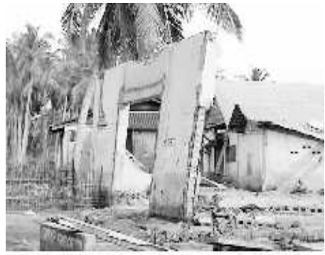
Once working offices, reduced to rubble.
