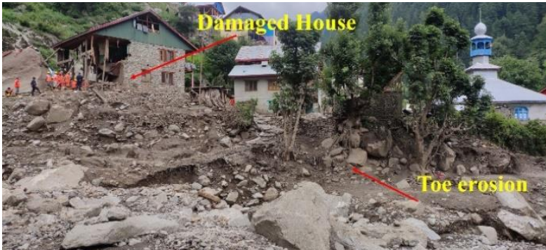
Photo 5. Damaged house and toe erosion
