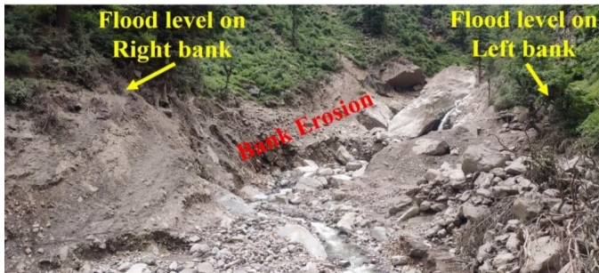
Photo 1. Flood level and bank erosion along Malo Rar Nala.
