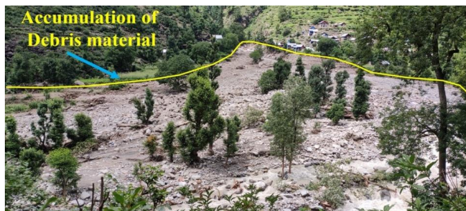
Photo 3. Debris deposited as a fan shape near the confluence of Malo Rar and Nanth Streams.
