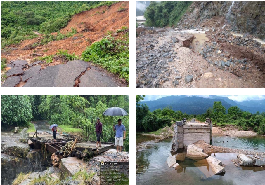
Fig 1B: Specimen photographs of eroded section of roads and bridges (Sources: DDMA, SWKH).
