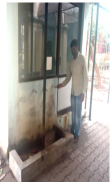
Figure 19: Drinking water facility
