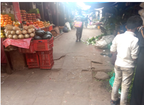
Figure 6: Narrow uneven ramp along the pedestrian way
