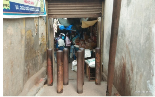
Figure 3: Stone posts on West gate
