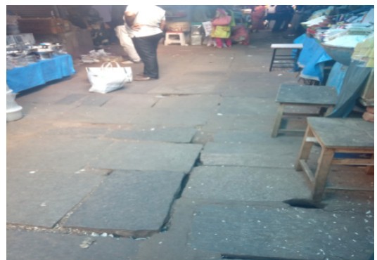
Figure 7: Uneven surface along the pedestrian way
