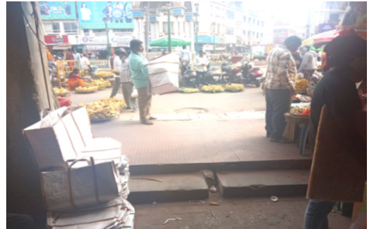
Figure 5: Steps without ramp on gate towards Dufferin Clock Tower
