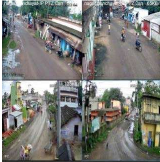
CCTV installation at all major public places.
